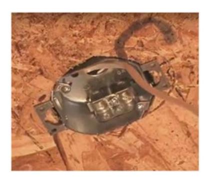
Note: shows installation in process, prior to addition of fasteners and sealant/expanding foam.
